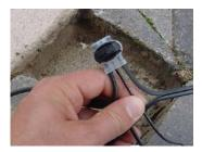
making sure that is it pushed all the way to the back. Finally take the black wire from a light and place it in the center hole, pushing it to the back of the connector. The connector should have 3 wires in it.
